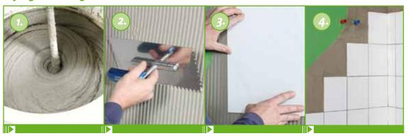
Put 6I of clean potable water into a clean mixing vessel, then add the powder in portions to the liquid while continually mixing with a slow rotating mechanical stirrer.
