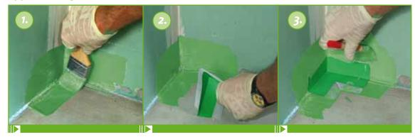
Apply a covering coat of KÖSTER BD 50 to the area in the inside corner where the KÖSTER BD Inside corner is going to be installed approx 10 cm up onto the wall and 10 cm onto the floor.
