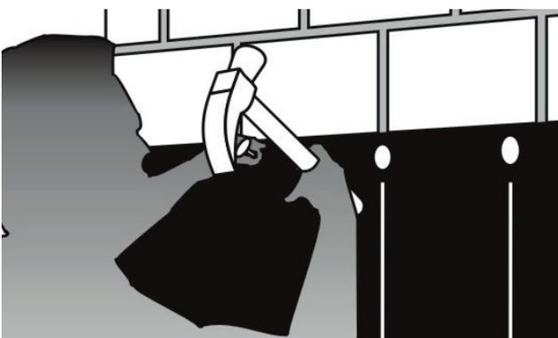
The upper edge of the membrane is fixed in position mechanically. Use large headed nails to fix the membrane in position.
